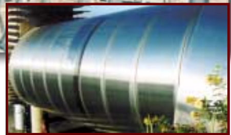
Aeroporto Fortaleza, Fortaleza, Brazil Architect: Claudio Silva, 1997 Stainless steel panels bonded to steel frame.
