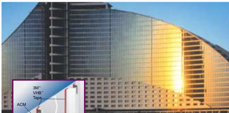
Jumeirah Beach Hotel, Dubai, UAE Curtain wall design: Schmidlin AG, 1998 Aluminum panels bonded to steel stiffeners.
